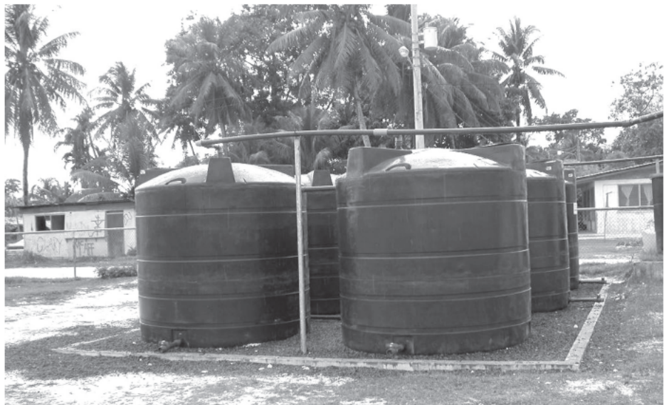
Rain catchment system at an elementary school on the island of Peleliu in the Republic of Palau.
